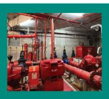
In support of our tenant, we completed a water saving project at 4 Pandan Avenue, Singapore in January 2023. This project involved the upgrade of the sprinkler pipeline and installation of a pressure relief valve that enabled the recycling of water which would otherwise have been drained off during the weekly sprinkler system testing. This project resulted in an estimated 80% reduction (2,900 CuM) in water consumption which translates to \$\$7,950 in savings annually<sup>16</sup>.
